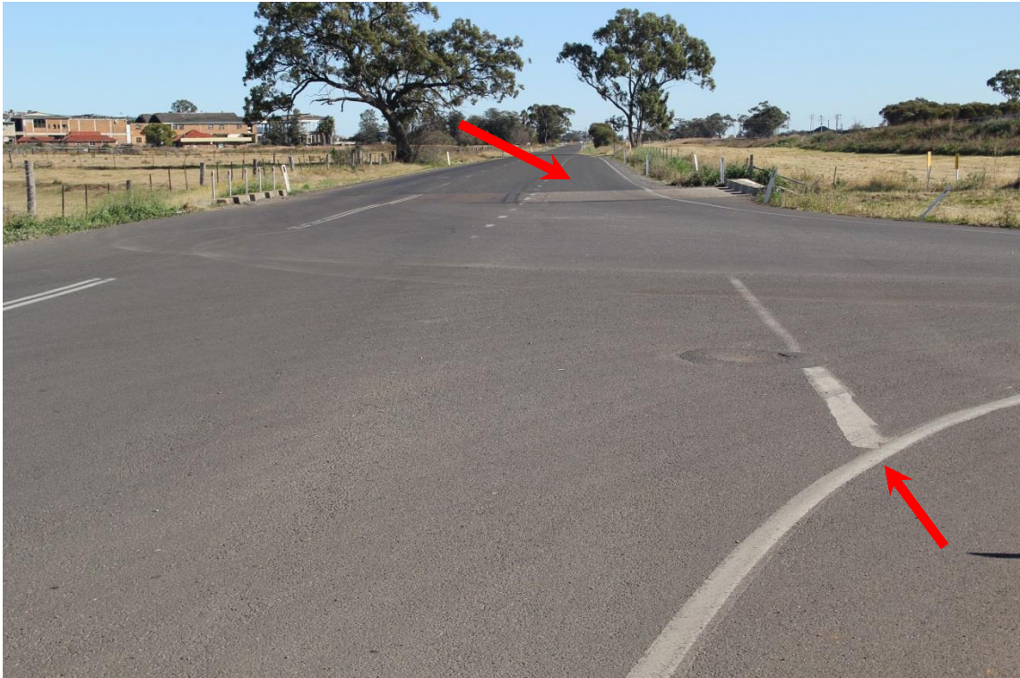
Photograph 9: West Along Quia Road from Farrar Road (Ross Road) Intersection
