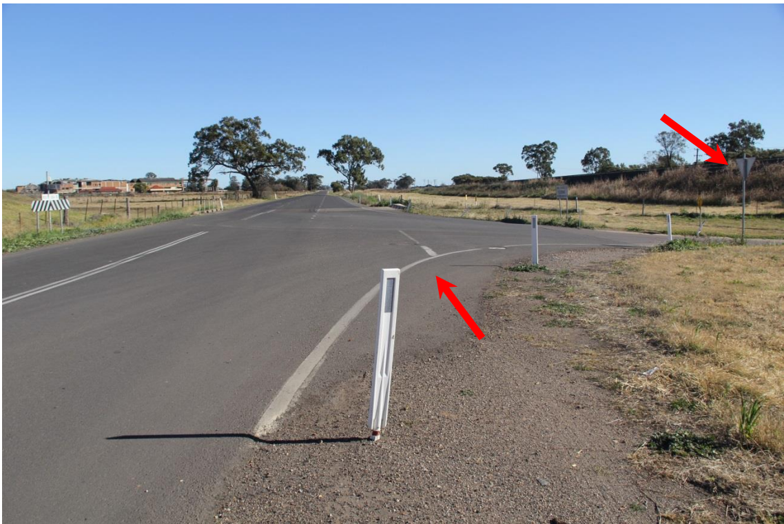
Conflicting non-standard "stop" line and "give way" sign on Quia Road.
