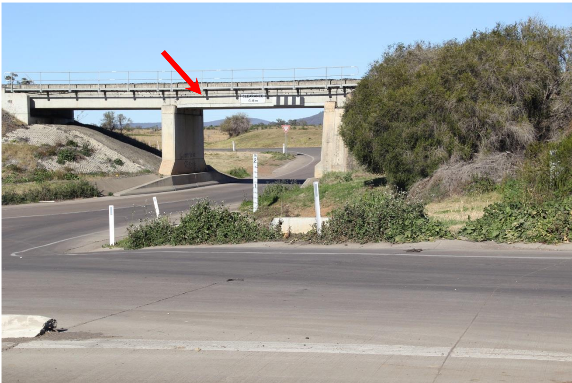
Photograph 8: West Along Quia Road to Railway Underpass
