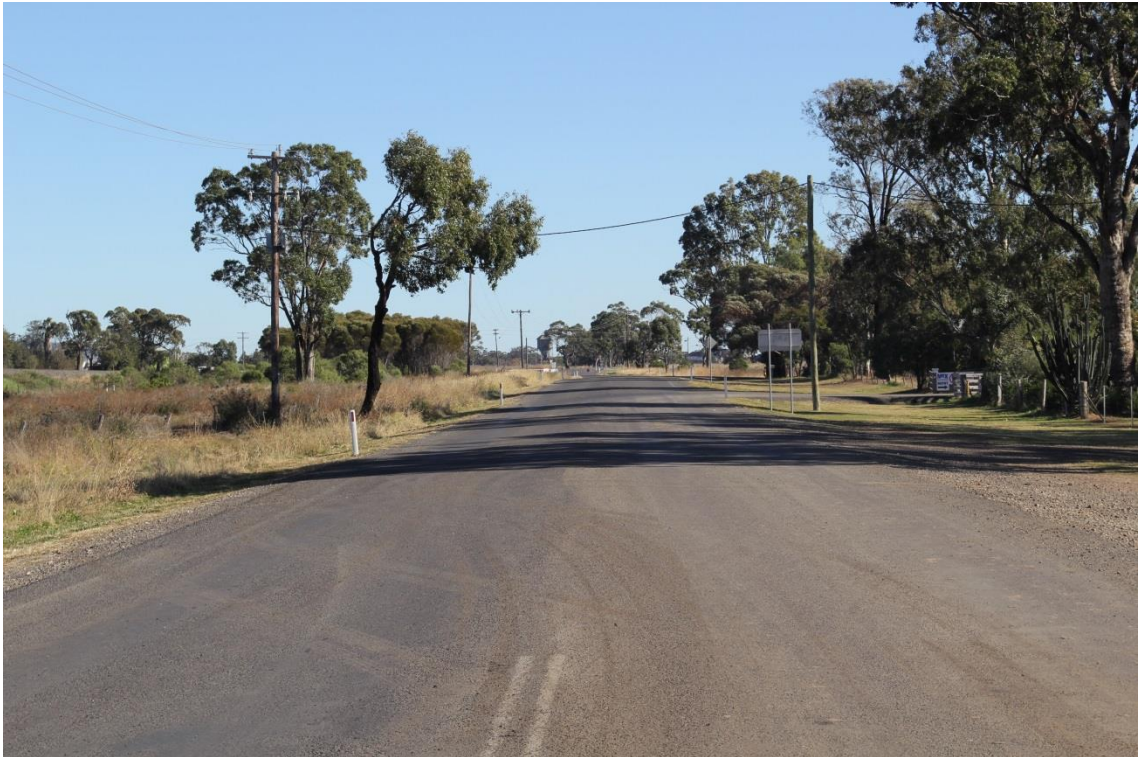
Photograph 12: West Along Torrens Road to CHPP Gates
