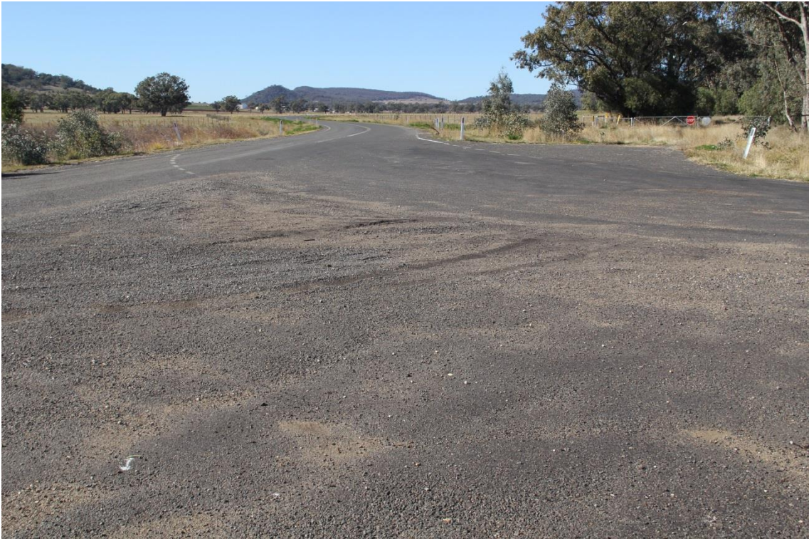
Photograph 3: Intersection of Coccooboonah Lane and Sunnyside Access Looking East
