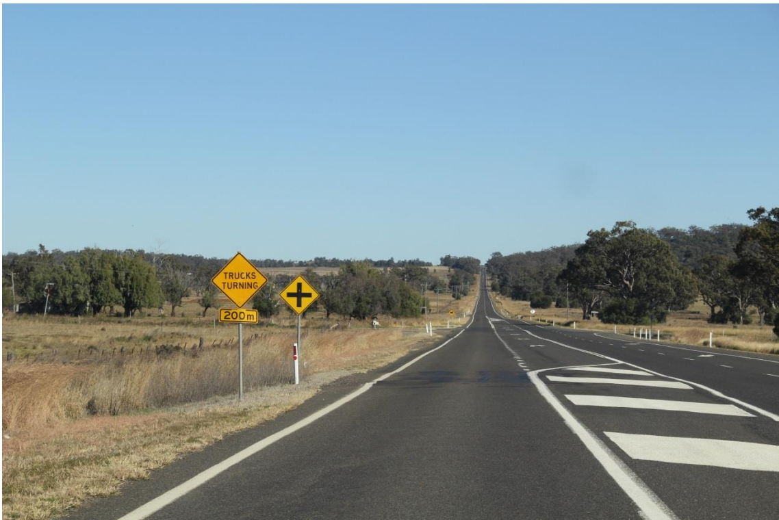
Photograph 5: Approaching Coochoonah Lane on Oxley Highway from Gunnedah
