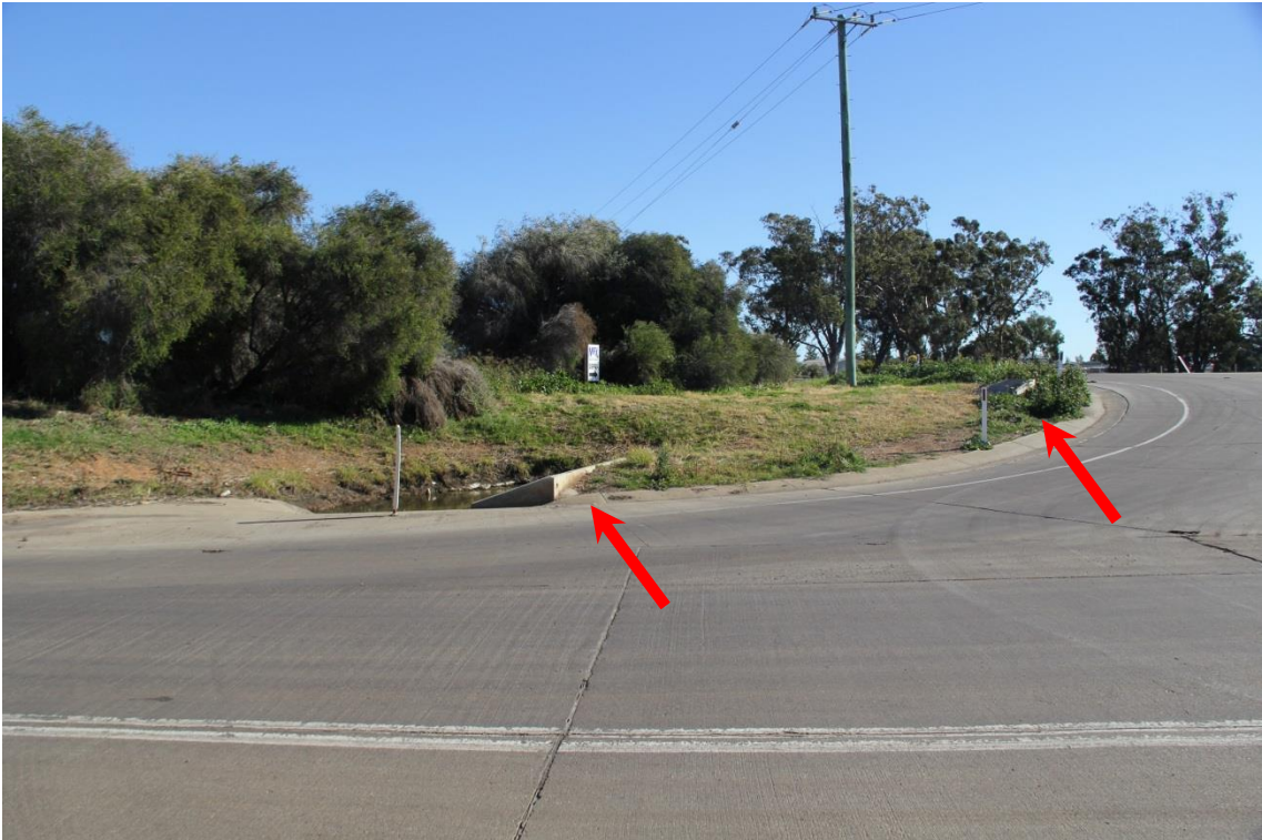
Photograph 11: Intersection of Quia Road and Torrens Road
